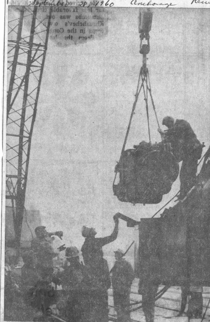
A PILE HAMMER is set onto the back of the unloading crane at the city dock to counterbalance the load while lifting four new cranes from a barge. The cranes, two 40-ton and two 7 1/2-ton, arrived yesterday from Seattle. They were shipped by Northland Freight Lines.
