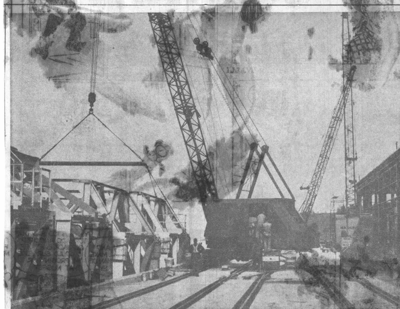
GANTRY CRANES ARRIVE — A crane unloads four bases — called gantries — from a barge at the Port of Anchorage dock. The giant bases will carry two 40-ton and two 7.5-ton cranes which will handle cargo at
