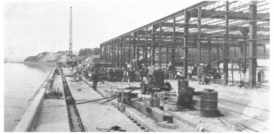
Looking northward along face of dock. Width of apron from rail to side of transit shed is fifty feet. Huge gantry cranes will straddle a double-rail track to expedite the handling of cargo from railroad cars directly to ships' holds.
