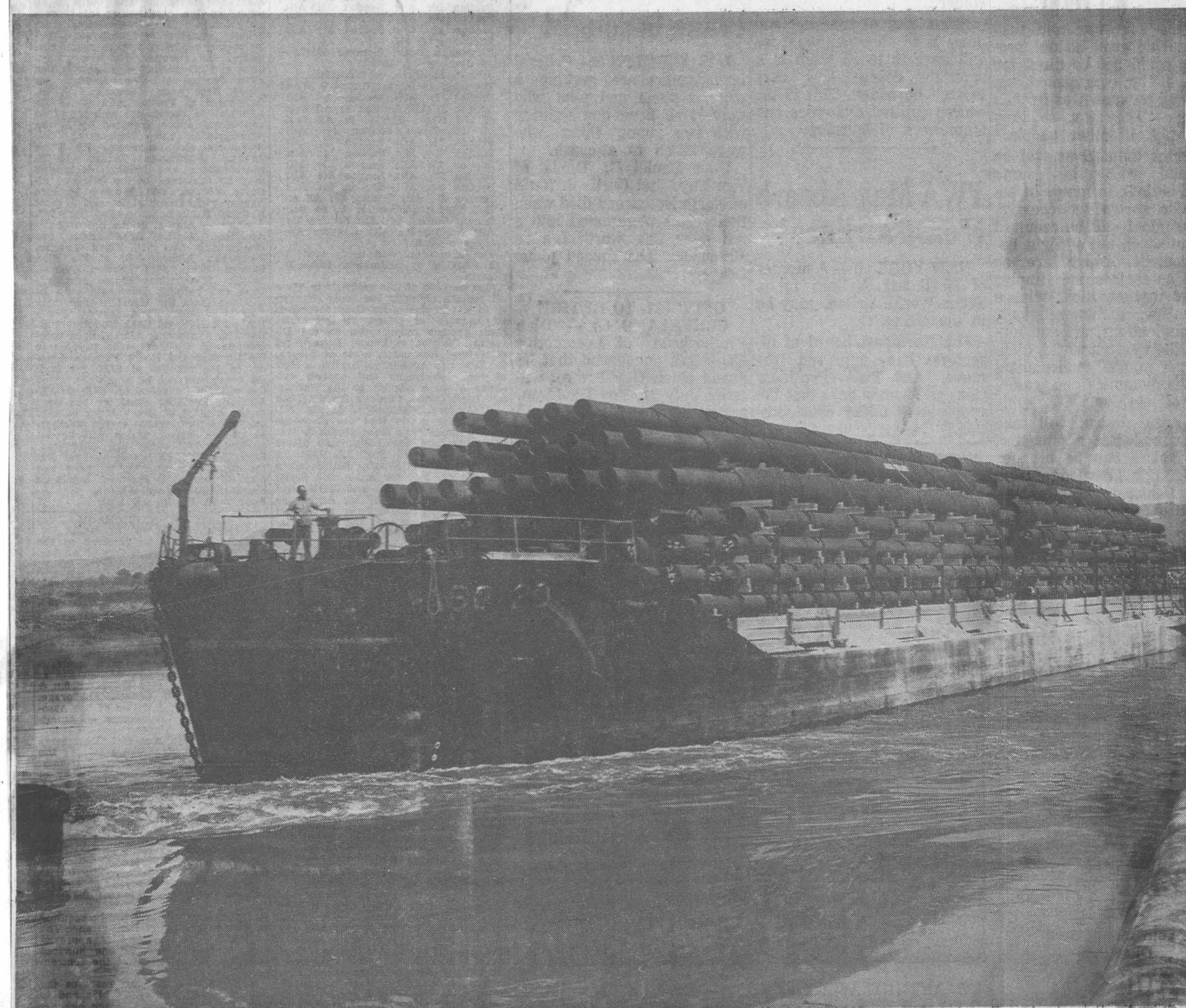
SIX MILES OF PILING — A Kaiser Steel barge loaded with 2,200 tons of piles for the dock arrived here recently. Over 400 lengths of the pipe of several diameters would stretch about 32,000 feet if laid end to end. A total of 1,144 piles are being driven, equalling about 80,000 linear feet. The city's consulting engineer on the project is Tippetts-Abbett-McCarthy-Stratton. General contractor is De Long Corp. The pile and concrete form work is being done by M. B. Gilbrough Co., and the concrete work by Anchorage Sand and Gravel.
