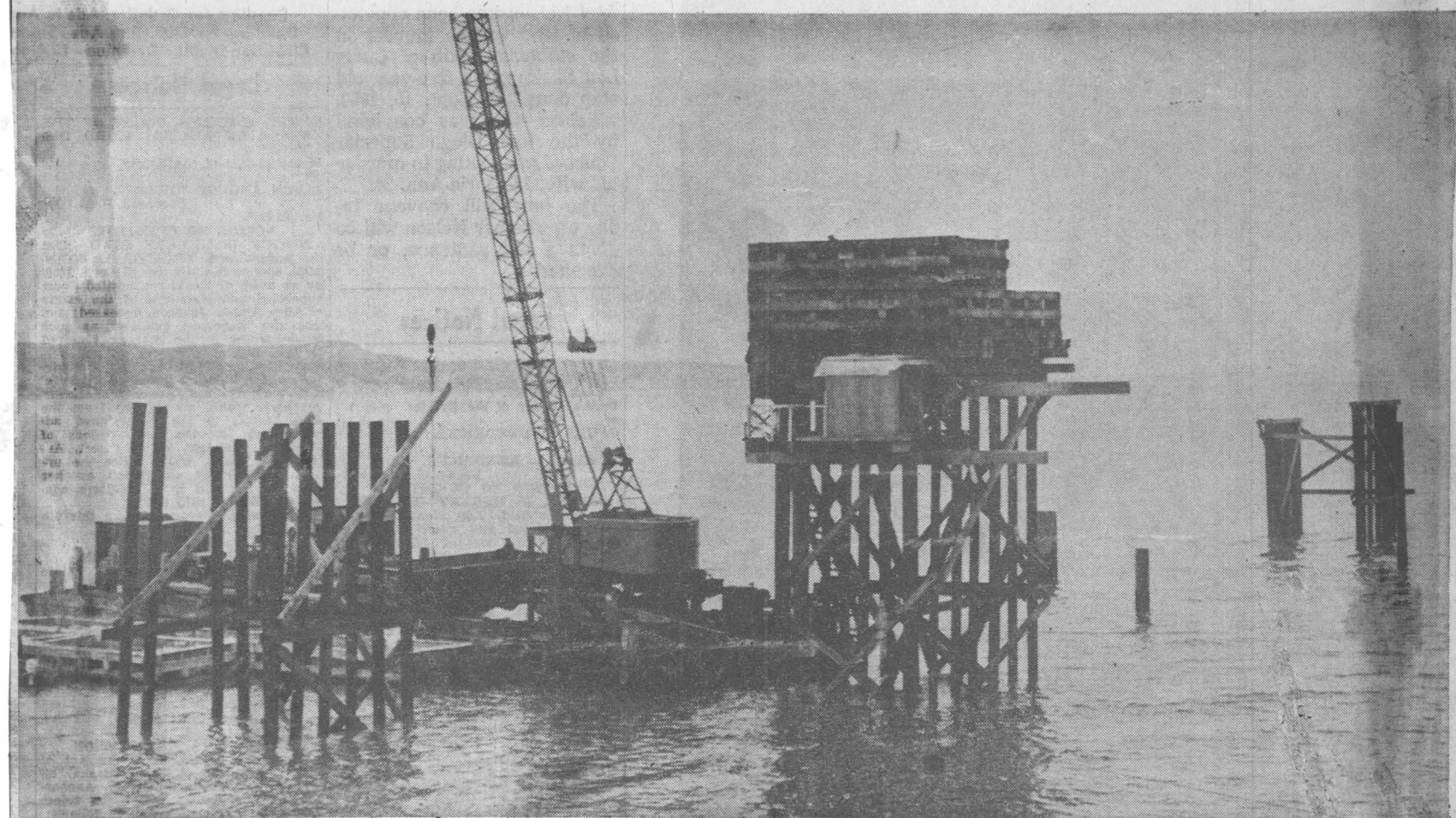
PORT PENTHOUSE — Apparently misplaced, a structure similar to this will rise this week in the waters off Anchorage's $8,000,000 port, now abuilding. The complex of pilings and huge boxes is used to load test pilings for support of the 500 by 300 foot deck.
