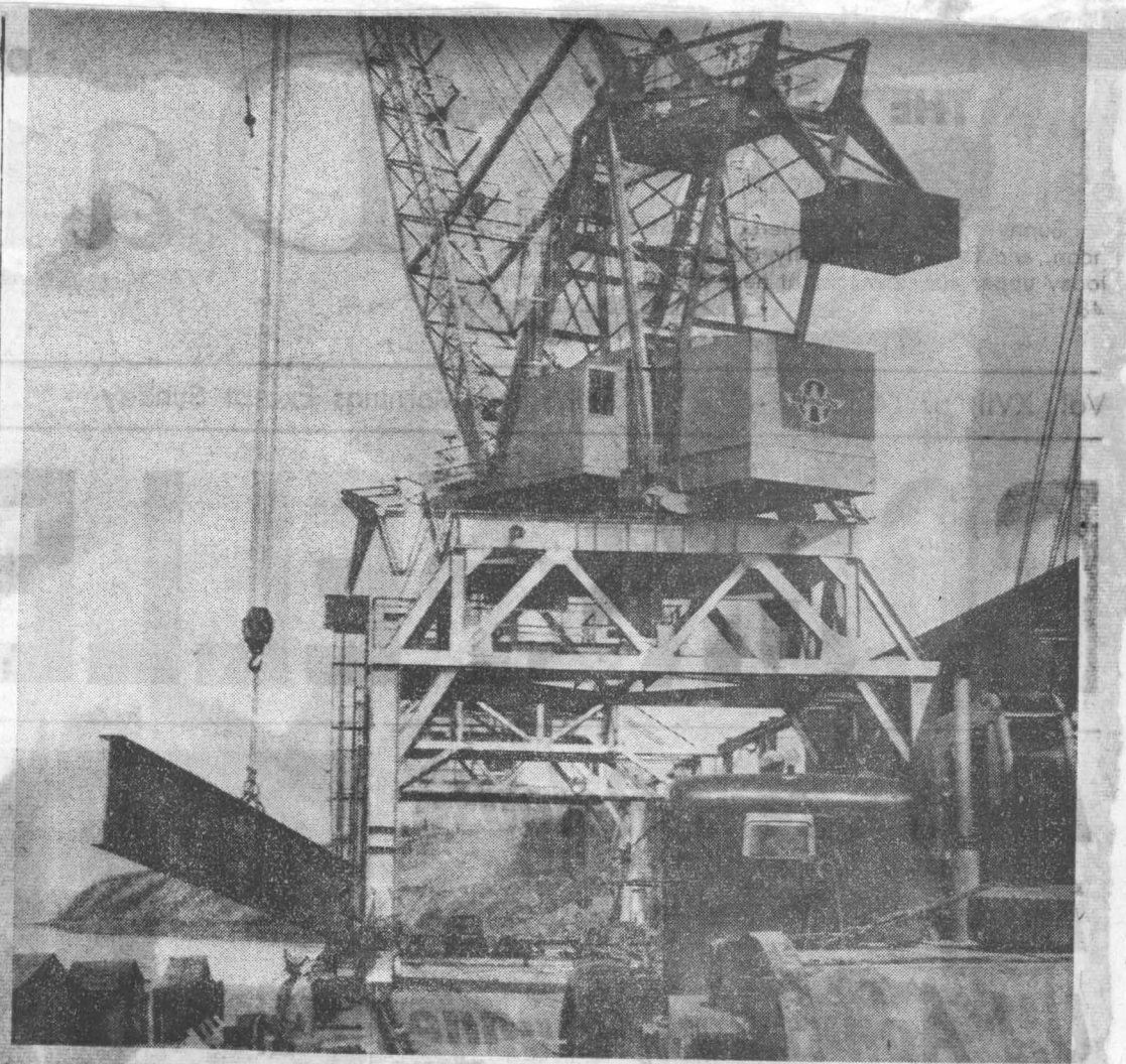
GANTRY CRANES at Port of Anchorage lift steel spans to waiting truck for the Matanuska-Knik crossing. Barge load was one of 700 tons out of 3,000-ton total for the bridges. Port Director E. N. Harned reports the total length of vessels at port now is 1,058 feet, a new record. (Daily News Photo)
