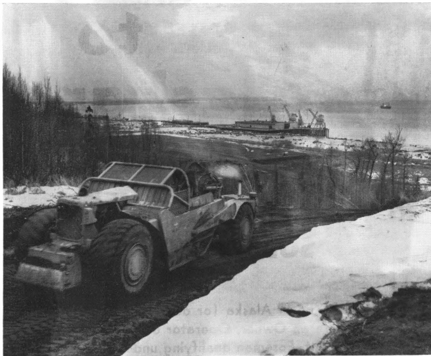
PORT EXPANSION —M-B Contracting Company equipment (Caterpillar 580) is shown at dock expansion work being done as a $150,000 emergency project by the U. S. Army Corps of Engineers. Anchorage port facilities were not destroyed by the Good Friday earthquake-tsunami waves as were Seward and Valdez. A staging area and new access was provided under the engineer program in addition to dock repairs.
