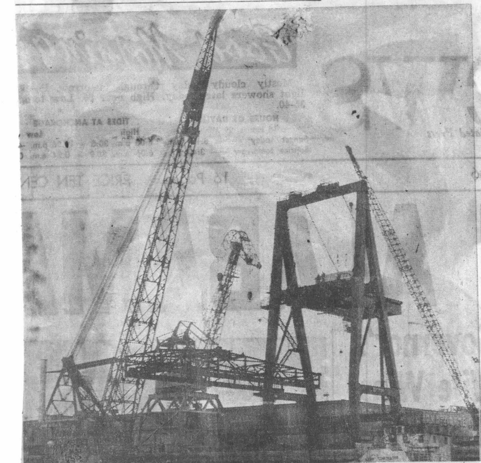
33 TONS OF METAL swing through the air as boom is hoisted into place on Sea-Land's giant crane at the Port of Anchorage municipal terminal yesterday. A giant derrick barge, capable of lifting up to 250 tons, was brought into Anchorage for the job. View of the operation is from the deck of the Elsie Foss, a small tug that stood by while the work was being done. (Daily News photo)
