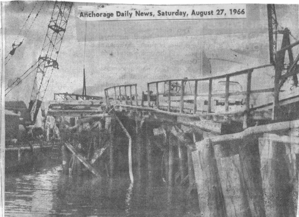
COMING DOWN is the entire front of the military's Ocean Dock in Anchorage's port area. The dock is considered a navigational hazard because of the extensive damage it suffered in the 1964 earthquake. About 2,000 square feet of the
