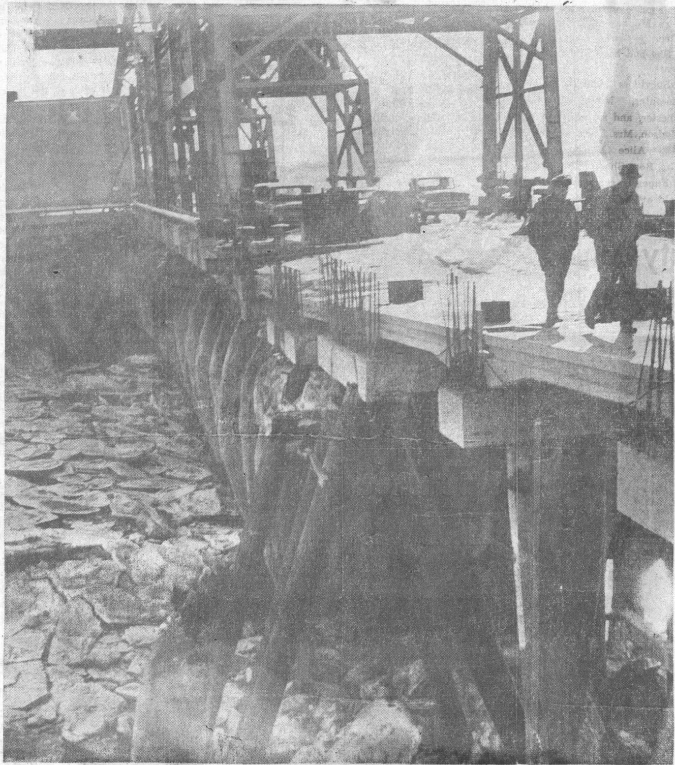
INSPECTORS STRIDE toward the northern end of dock extension past broken concrete pads topping support piling. The piling cap in center of the picture with cluster of reinforcing rod thrusting upward is one of
