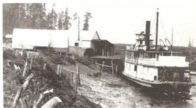
LATHROP DOCK (Anchorage Port Facilities — 1915)
