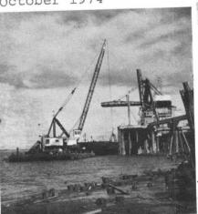
There's a disturbing operation going on at the Port of Anchorage. General Construction Company of Seattle is busy on a \$384,000 contract awarded by the Alaska District, Corps of Engineers, dredging the harbor. What they are disturbing, though, is useless and troublesome silt and shoaled material which builds up on the waterfront each year. The contractor will dredge to 35 ft. below mean lower
