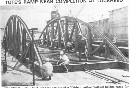
SEATTLE — The first 100-foot section of a 300-foot roll-on/roll-off bridge ramp for Totem Ocean Trailer Express (TOTE), takes shape at Lockheed Yard in Seattle. Complete ramp assemblies will be in place at pier facilities in Anchorage and Seattle in late August. Five ramps are to be built. They will be used by the "Great Land" in the Seattle-Anchorage trade. The "Great Land" is the first all ro/ro trailership to be utilized in this trade. (Photo by Jim Davis)
