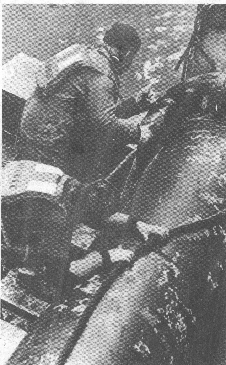
The drag pipe, capable of reaching 75 feet into Cook Inlet waters to clear shoal.
