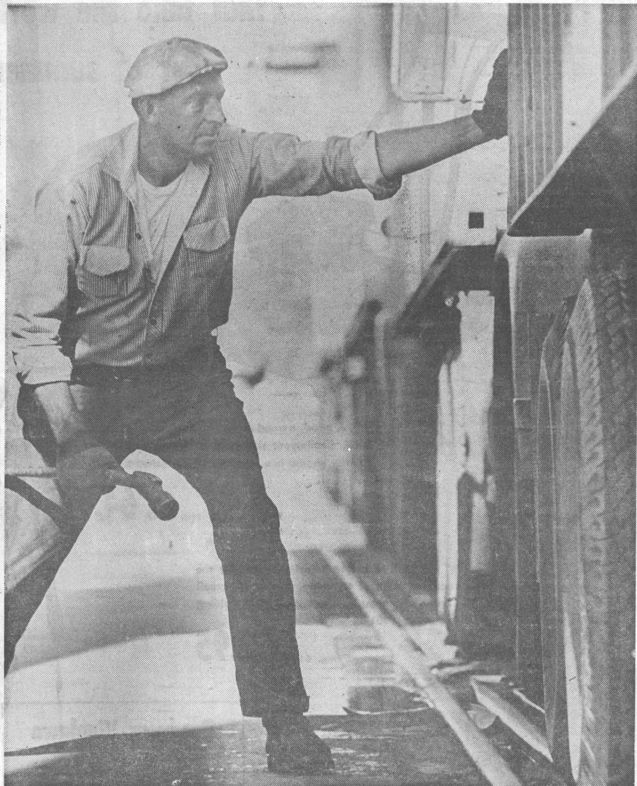
Tom Vitts eases an empty Sea-Land container onto the trailer on which it'll be hauled to the Sea-Land "pit" and dispatched to some point in Alaska. The container operation allows a ship to be unloaded and loaded simultaneously, helping to cut dock time in half.
