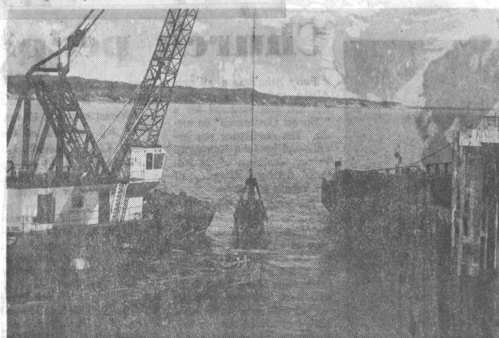
General Construction Co. dredging at City Dock
