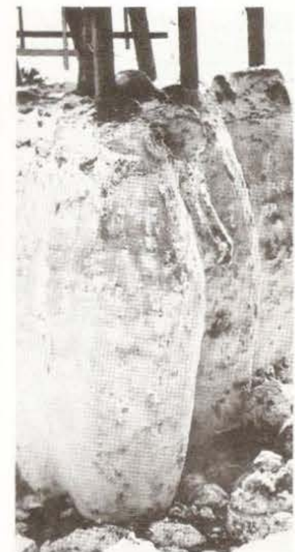
Floe ice 4 ft (1.2 m) thick carried by some of the strongest tidal currents in the world striking the pipe piles was just one of the unique conditions faced by TAMS designers. Another was the 20-ft (6.1-m) thick ice buildup under the wharf adding to the weight and uplift applied to piles with 70-ft (20-m) unsupported lengths.
