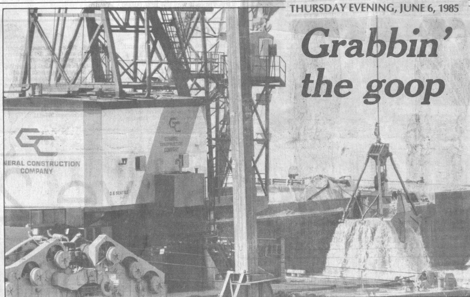
Mud spills from the maw of a giant crane gouging out a 2,900-foot-long, 150-foot-wide trench in the Port of Anchorage
