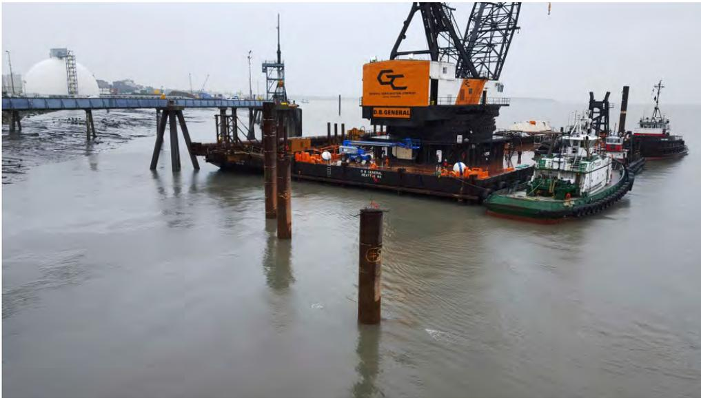
Figure 2. KIWC Barge-mounted 700-Ton Derrick Crane – DB General.
