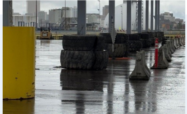
Equipment tire column base protection installed
