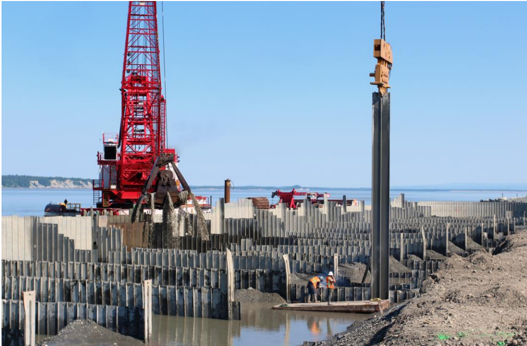
NES1 Sheet Pile Removal
