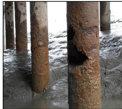
Anchorage spends $3 million to repair about 100 severely corroded wharf piles each year. The port has a total of 1,423 wharf piles.
