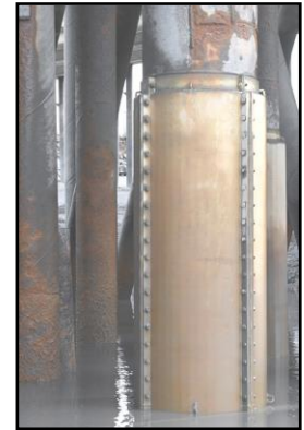
Recently jacketed pile.
