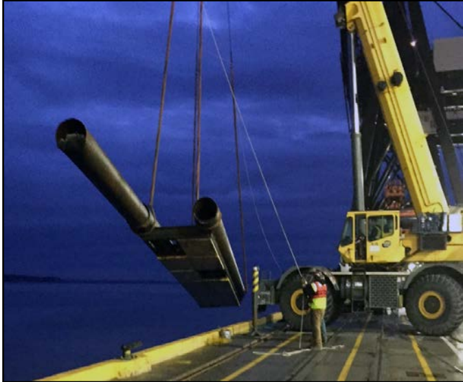
Crane lifts 57,000-pound dock fender out of ship berth at 2 AM on June 27, 2017.
