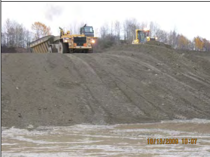
QAP staging fill in center stack.
