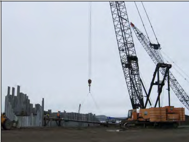
North pad, South end at departure – Orange 2500 picks gangway, lifts onto support brace, 4100w Black tip carries man basket to cell 21 for tail wall brace installation
