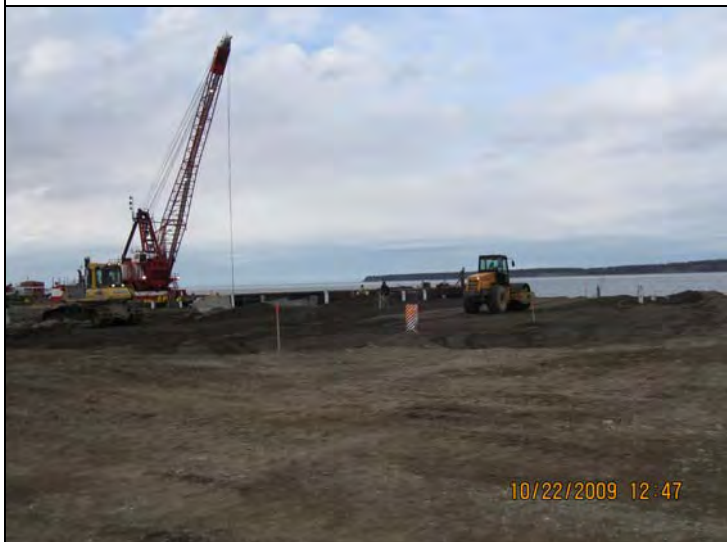
Grading and rolling cells 44-50.
