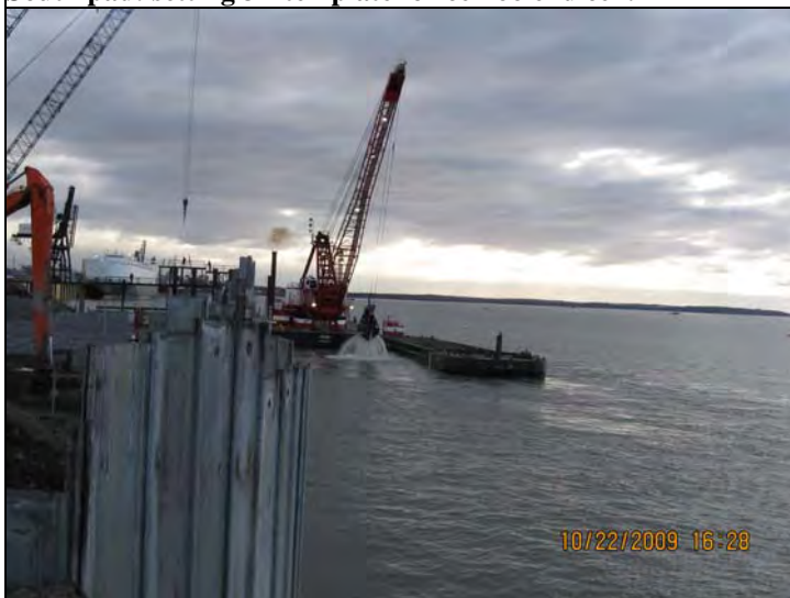
Manson dredging off N. Extension cells.
