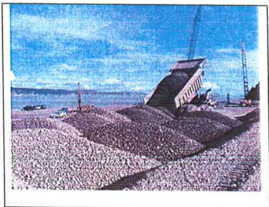
Figure 1 Vibrocompaction fill
