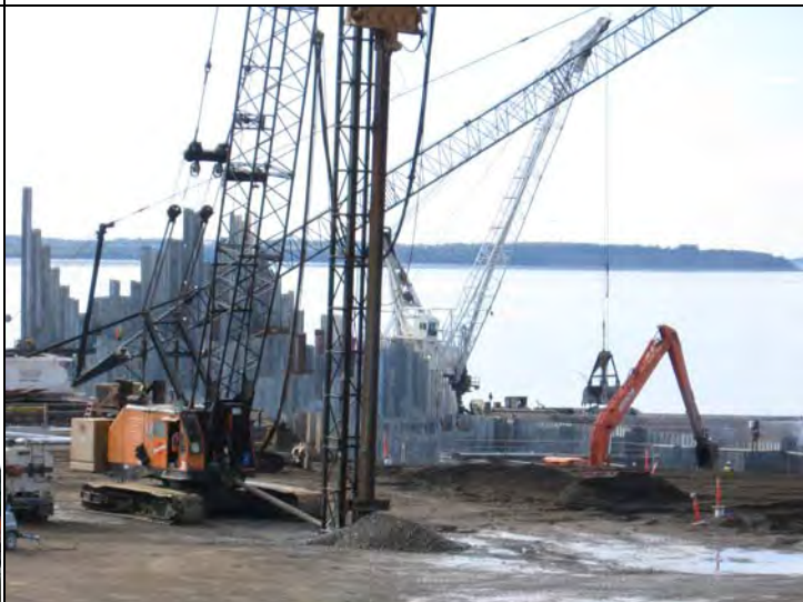
North Pad, North end at departure – 4000w Vibracompactor working East of cell 15 w/ Volvo Loader and QAP water truck assisting; cell filling operations continue in background
