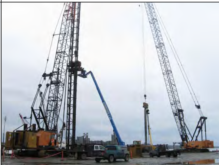
North Pad, North end at departure – 4000w Vibracompactor stopped for a temperature check of its Ape 200-6 vibratory hammer while 2500 Orange pauses w/ raised sheet from tail wall J (10S) to allow crew to affix safety cable to hammer prior to releasing sheet from hammer jaws, laying on sheet on pad
