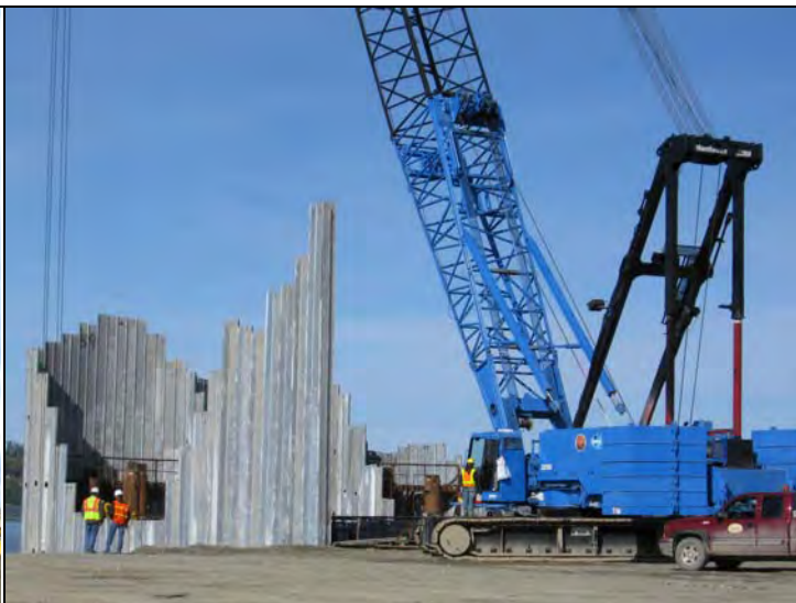
South pad, South end at departure – 2500 Blue positions Ape 200-6 to drive sheets tail wall BE, 4100w Orange tip drives sheets tail wall AY w/ BSP SL30
