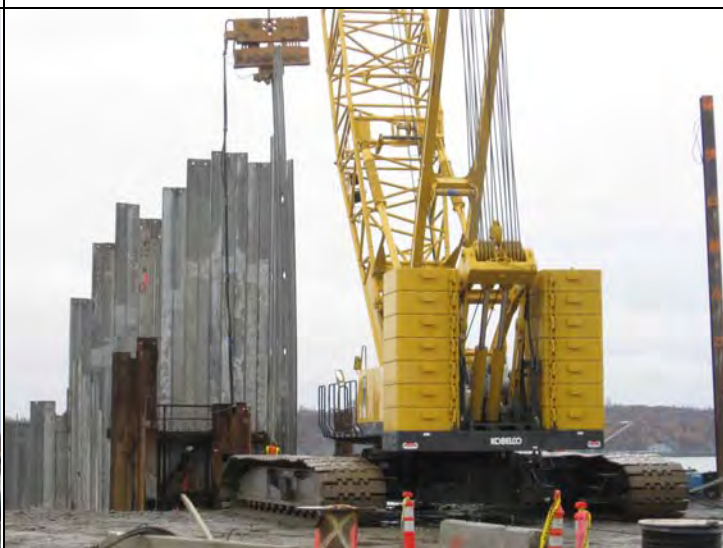
South pad, North end at departure – 2500 Yellow setting face sheets cell 39S w/ Ape 200-6; note skew of hammer/bend of sheets and long, uneven sheet drives; hard driving observed
