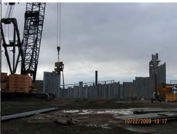
Driving out extended tail wall K.
