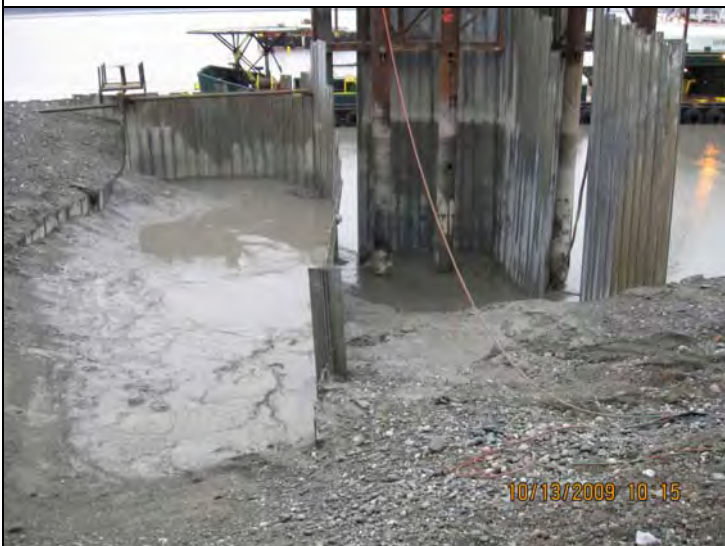
Note large differential fill between cells 12 & 13.
