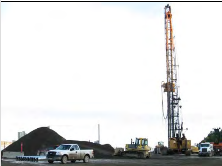
North Pad, North end upon arrival – 4000w Vibracompactor working East of cell 15 w/ Volvo Loader and QAP water truck assisting; 4100W Black tip idle in background, boom on ground; Komatsu 61PX fills cells ~15-22
