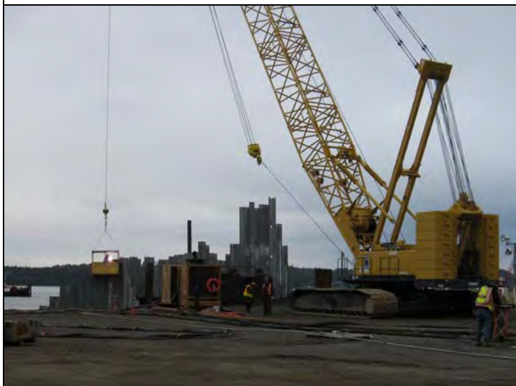
South pad, North End upon arrival – 2500 Yellow carries man basket/1 crew to cell 40 where crewman trims sheets, welds plates to sheets in attempt to stiffen – TWA surveyors right
