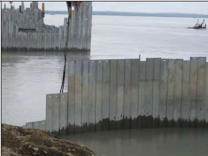
Wet Barge Berth – 2500 Yellow w/ JM 115 – After – Some progress made on 4 sheets shown, cutoff required on bent sheets to the north
