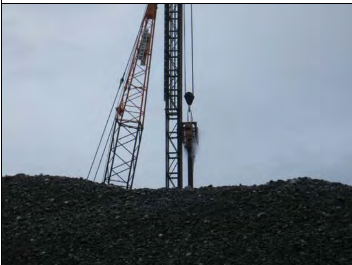
Steam and or water vapor obscure the Ape 200-6 vibratory hammer in a cloud of white mist atop the 4100w Vibracompaction crane
