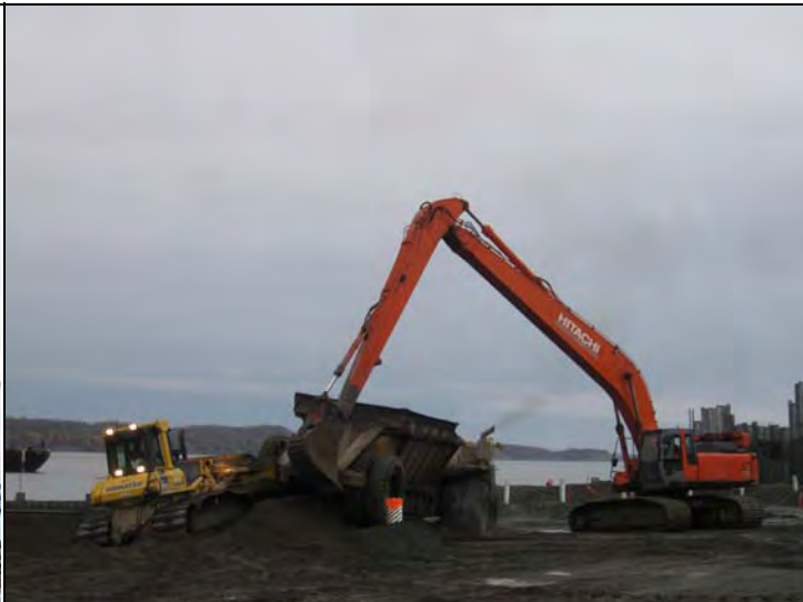
QAP Komatsu P61 bulldozer, Hitachi EX450 help free QAP 'Lizard' belly dump from 15 yards of freshly dumped fill during cell 21-27 area filling operations
