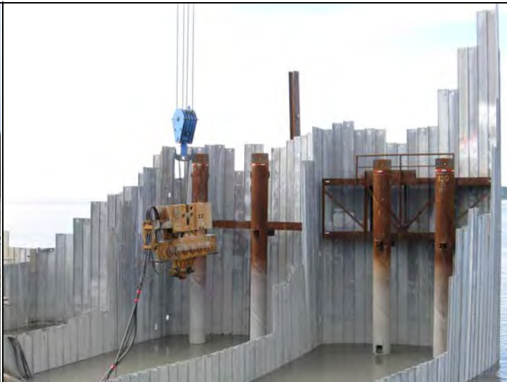
Ape 200-6 lifted out of flooded cell 38 where the hammer was partially immersed to allow for more rapid cooling
