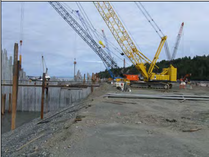
Sheet set down by 2500 Yellow after fitment & interlock interference issues prevent sheet installation
