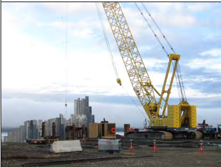
South pad, North End upon arrival – 2500 Yellow carries man basket/1 crew to cells 39/40 where crewman trims/weld sheets
