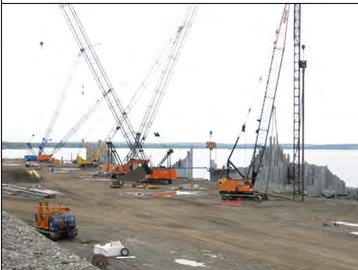
North pad, North End upon arrival – 4100w Black tip idle, crew work on BSP SL30 impact hammer, 4000w Vibracomp. Idle, Denali Drill rig idle
