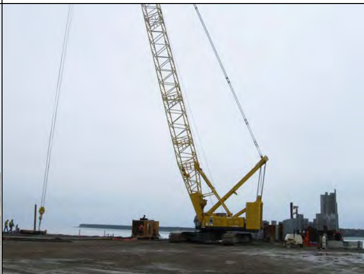
South pad, North End at departure – 2500 Yellow idle w/ Ape 200-6 on ground, crew 'cussing and discussing' failure to move sheets cell 40 despite add'l material welded to plates
