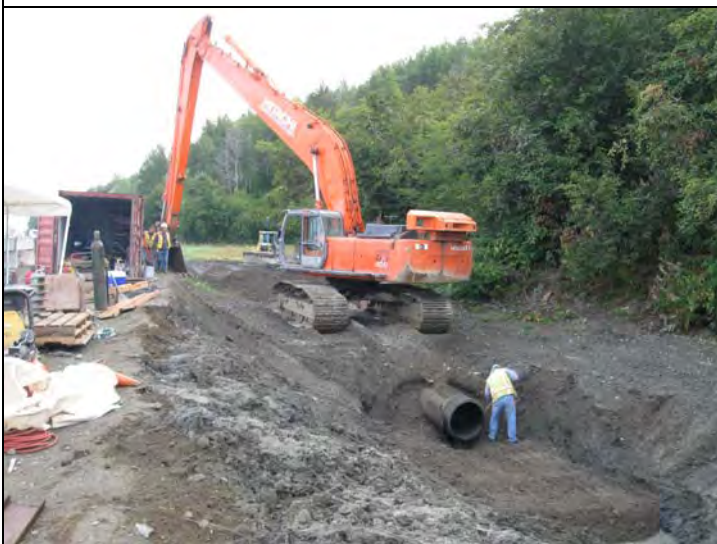
South Pad Drainage inlet – excavated, prior to compaction, density testing and cap/grate installation
