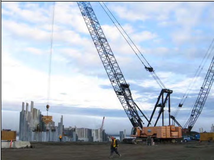
North pad, South End upon arrival – 2500 Orange driving sheets tail wall AB, 4100w Black tip idle in background
