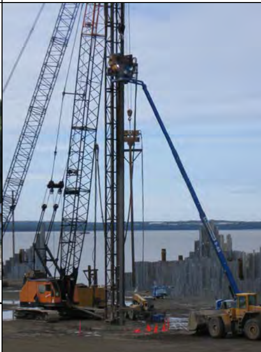
Ape 200-6 lifted out of flooded cell 38 where the hammer was partially immersed to allow for more rapid cooling
