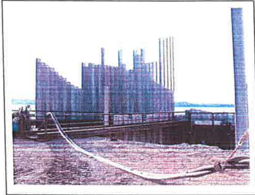
Figure 01 Sheet-Piles standing in place on the template at cell 24
