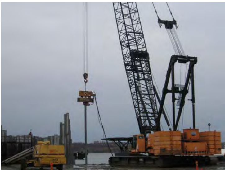
North Pad, North end upon arrival – 2500 Orange pulling sheet tail wall I (10N) w/ Ape 200-6 vibratory hammer
