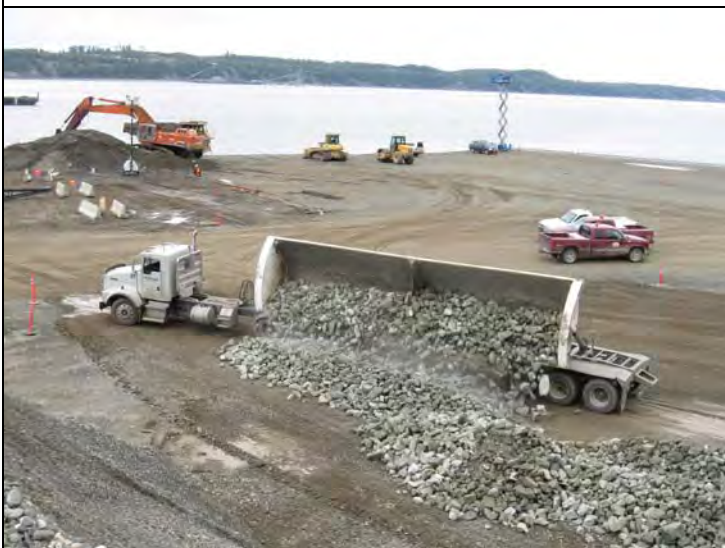
Tractor trailers w/ side dumps arrive w/ shot rock, form stockpile
