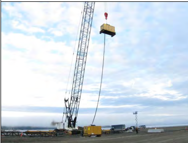
Wet Barge Berth upon arrival – 1500 White Lima moving JM 115 power pack
