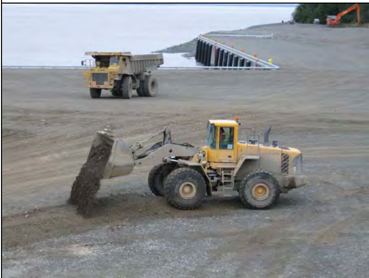
2 buckets+ fill removed from vibrocompaction fill stockpile and placed on ground by QAP loader
