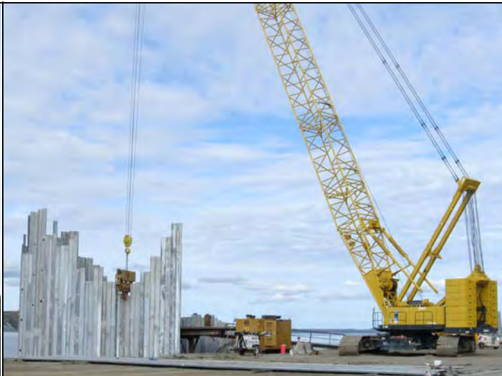
North Pad, South end at departure – 2500 Yellow drives tail wall AE sheets; 1500SC Lima returns Man Lift from from outside face cell 22 w/ crewman
