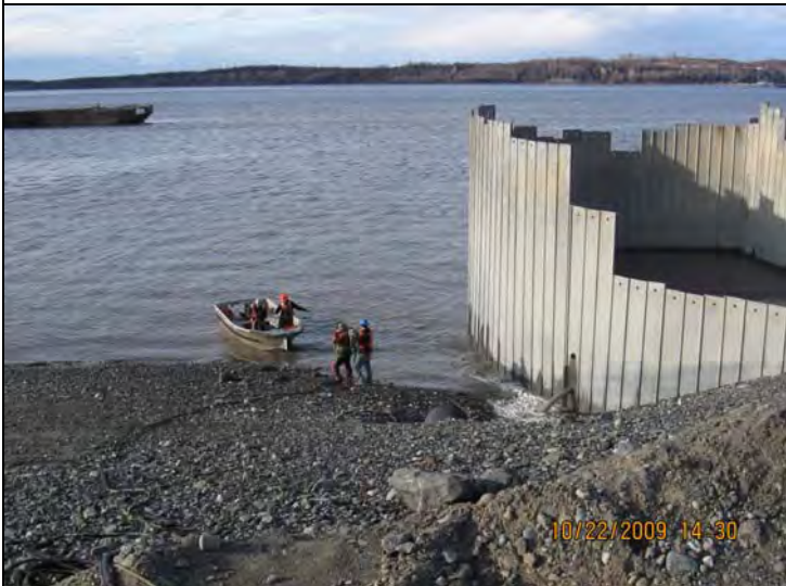
Global Offshore divers preparing to inspect WBB cells 36-38.
