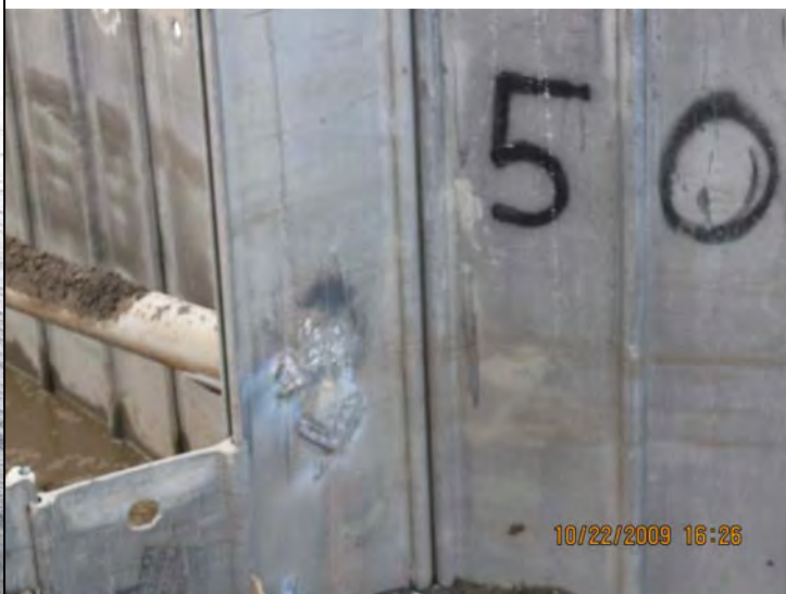
Coating repair on bracing welds cell 50.
