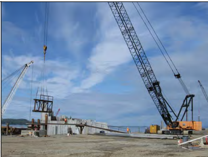
North Pad, South end at departure – Orange 2500 picking template to install at cell 28 face
