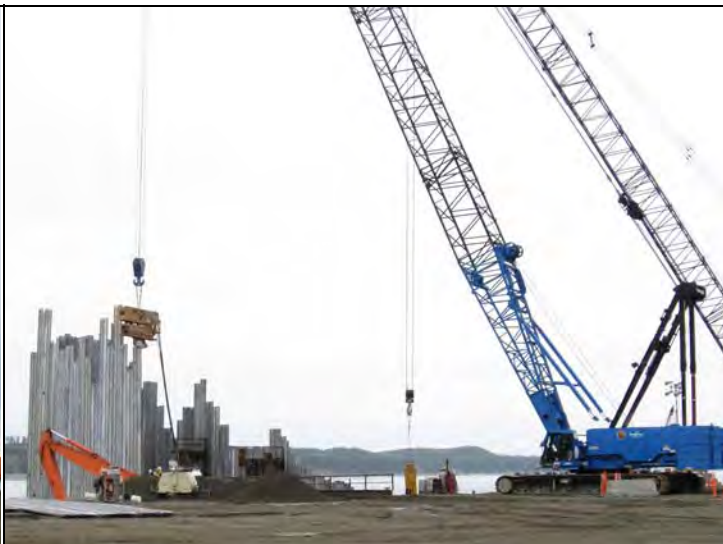
South pad, South end at departure – 2500 Blue drives sheets tail wall BE w/ Ape 200-6, 4100w Orange tip drives sheets tail wall BB w/ BSP SL30, Hitachi 450 excavates south of BE
