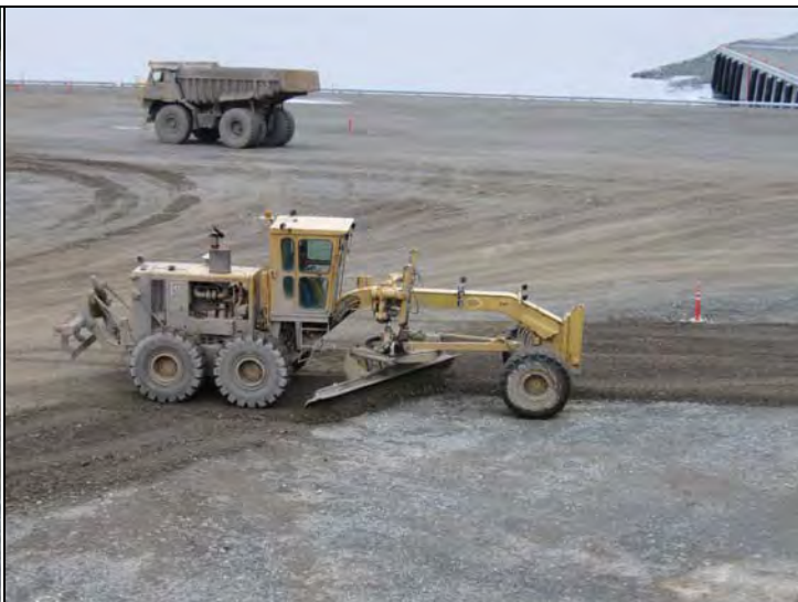
Grader fills holes and puddles and makes the approach more even
