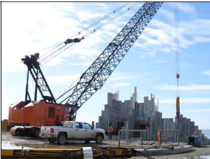
South pad, South end at departure – 4100w Black tip driving face sheets cell 56
