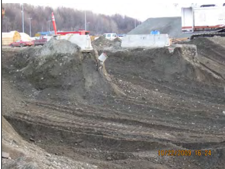
Inclinometers in cell 54 and 55 partially exposed by fill ramping.
