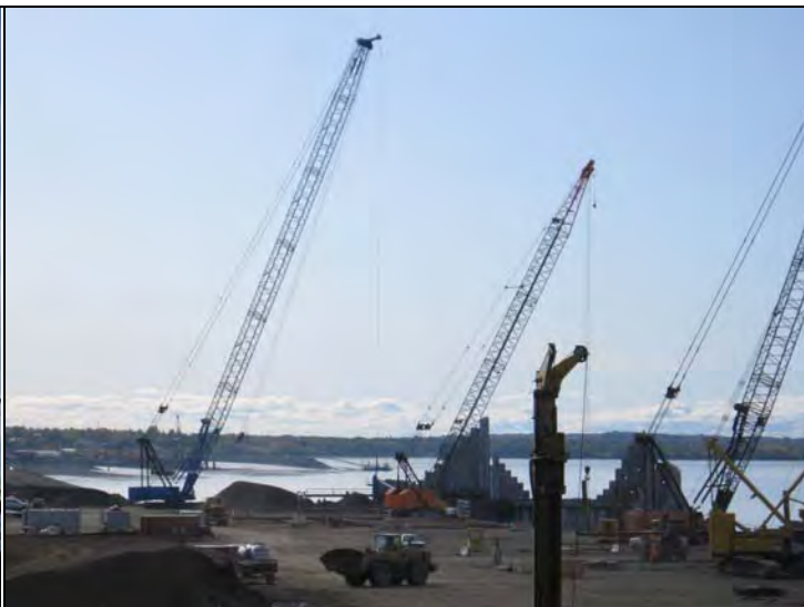
South pad, South end at departure – 2500 Blue stabs intermediate tail wall BG sheets while 4100w Orange tip drives sheets tail wall BD (cell 58/59)
