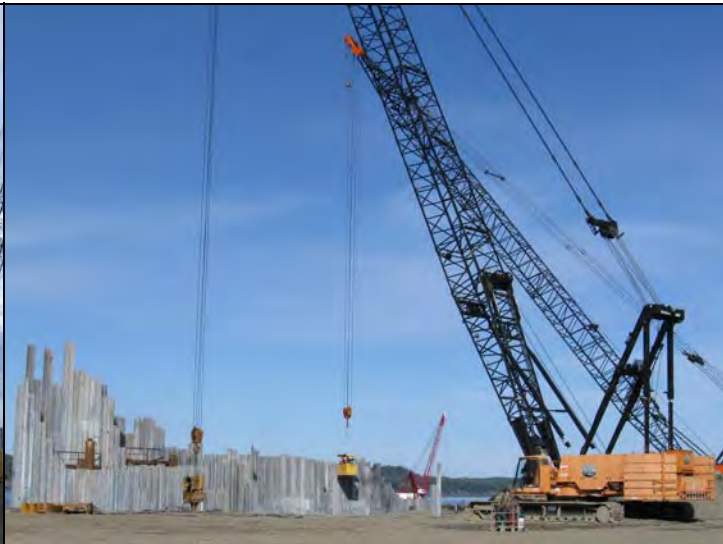
North pad, South end at departure – Orange 2500 drives sheets tail wall AB w/ Ape 200-4 & Pogo, 4100w Black tip carries man basket to cell 24 for Terracon to repair/connect sensor wiring
