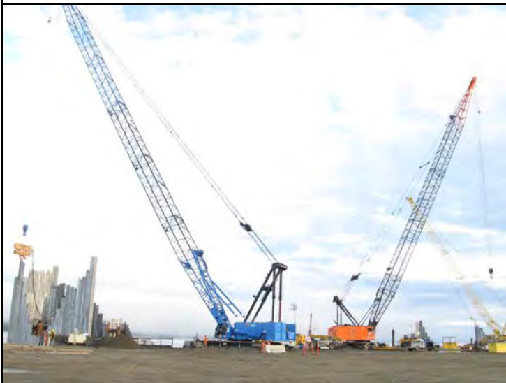
South pad, South end upon arrival – 2500 Blue idle w/ Ape 200-6 in position, 4100w Orange tip idle
