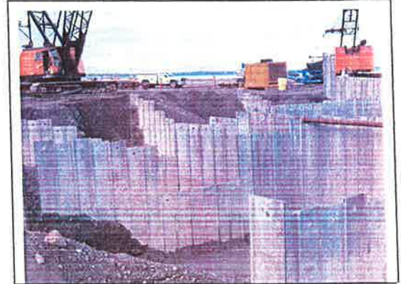
Figure 02 Preparing to drive tail piles
