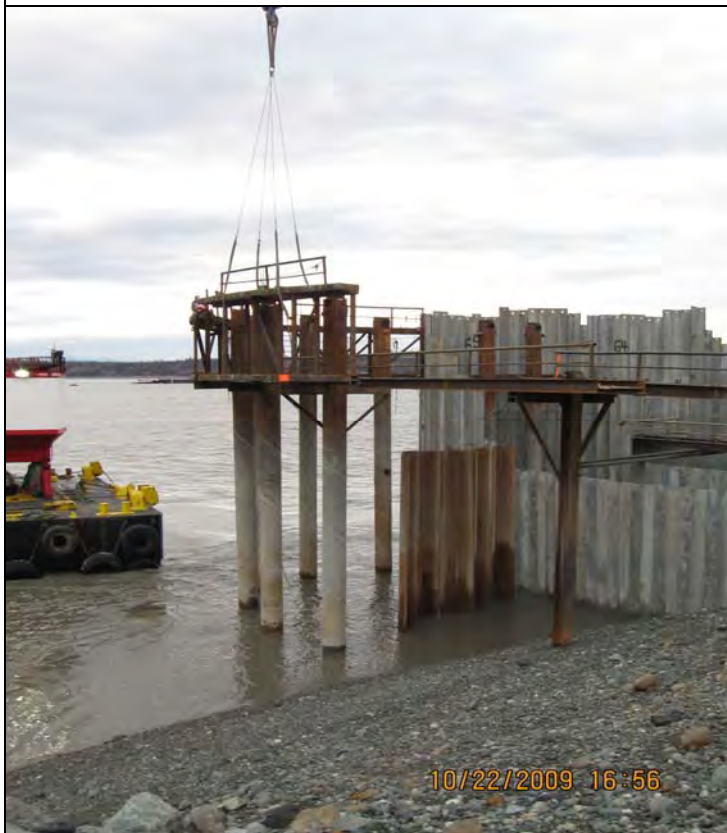
South pad: setting 3 rd template for cell 66 end cell.
