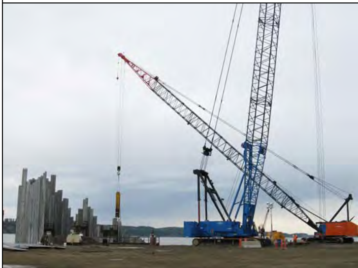
South pad, South end upon arrival – 2500 Blue idle, 4100w Orange tip w/ BSP SL30 impact hammer driving face sheets cells 56-57
