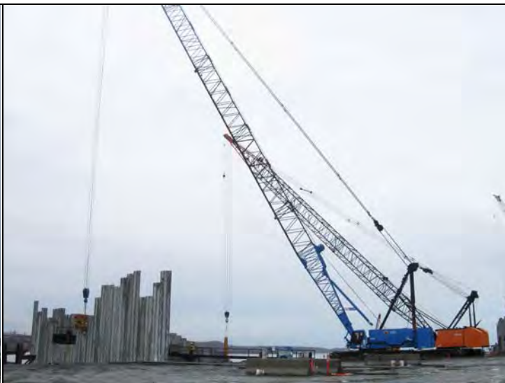
South pad, South end at departure – 2500 Blue 2500 Blue driving sheets tail wall BJ (cell 64s) w/ Ape 200-6; 4100w Orange tip idle atop tail wall BE (cells 59/60) w/ BSP SL30, bent sheet tip beneath hammer
