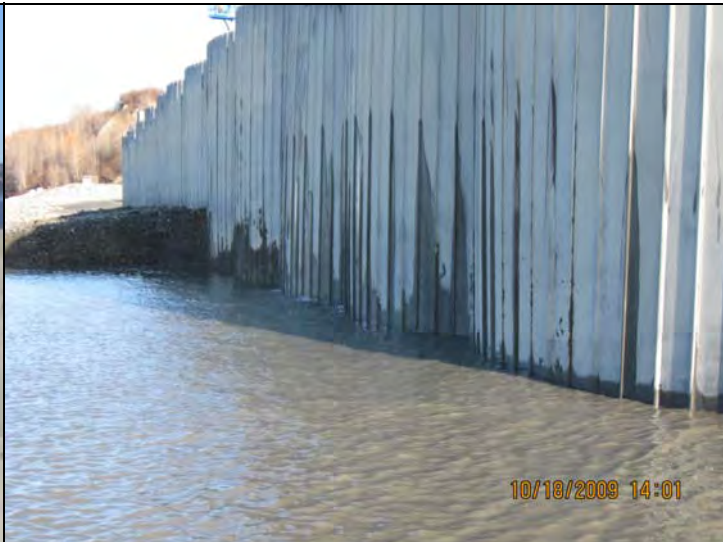
Wet Barge Berth cells 36-38 note the level of the water coming out through interlocks from the inside.
