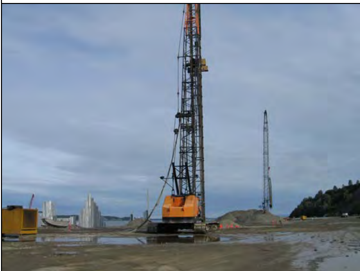
North Pad, North end & Wet Barge Berth upon arrival – 4000w Vibracompactor and White Sandstrom 'Lima' idle
