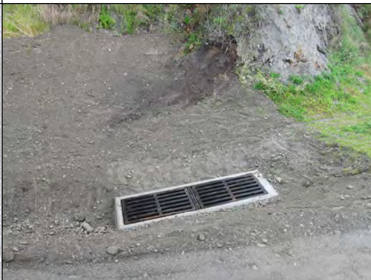
North Pad Drainage inlet – finished, covered up w/ cement cap and drainage grate installed
