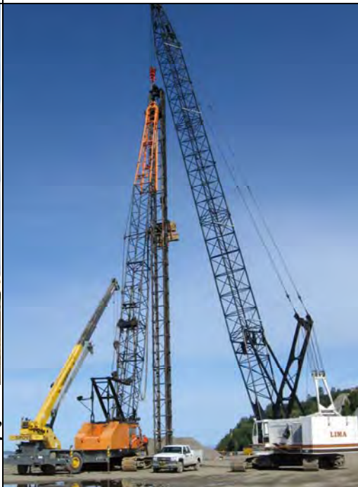
North pad, North End at departure – 4000w Vibe idle, repairs underway w/ 1500w Lima crane, Manlift
