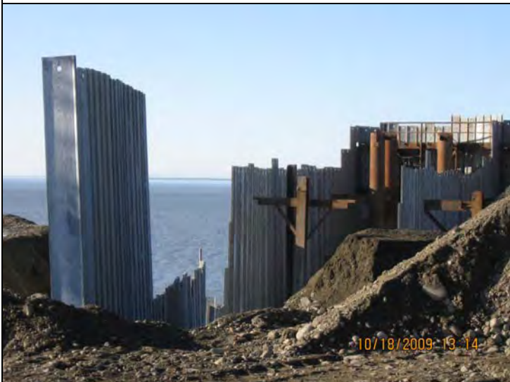
Extended tail wall BJ cell 64, note the lean.
