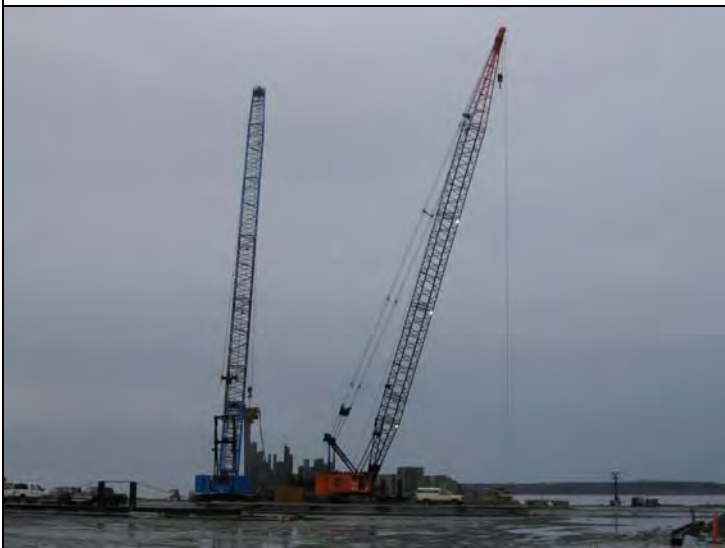
South pad, South end upon arrival – 2500 Blue setting face sheets tail wall BJ (cell 64s) w/ Ape 200-6; 4100w Orange tip carrying man lift to tail wall BE (cells 59/60) to trim sheets
