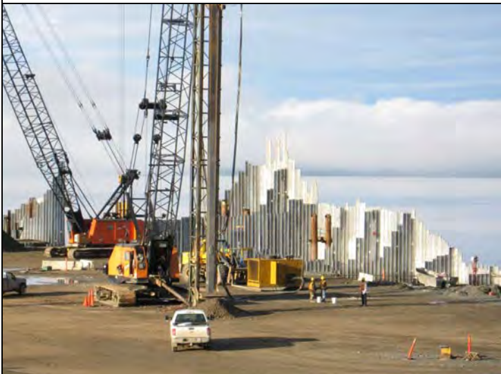
North pad, North End upon arrival – 4100w Black tip idle, crew work on JM 115 impact hammer, 4000w Vibracompactor active, Denali AF80 auger active
