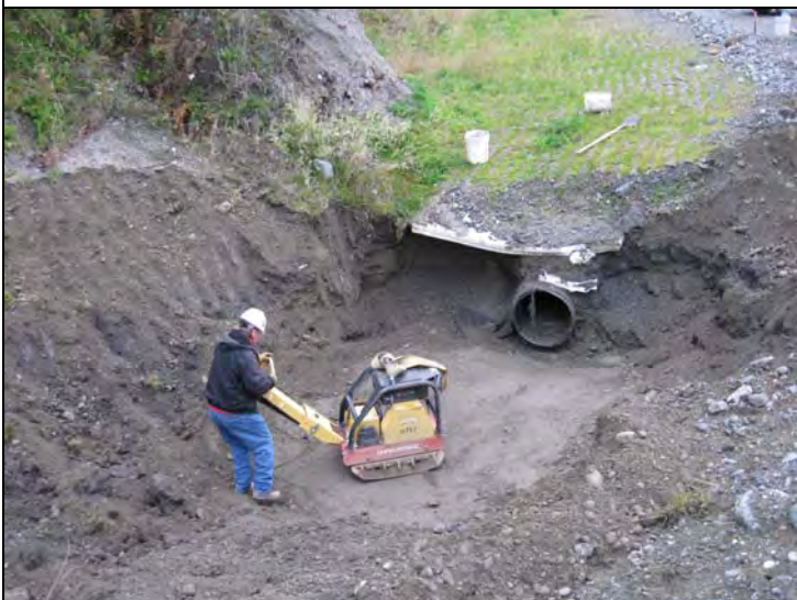
North Pad Drainage inlet – excavated, under compaction prior to density testing
