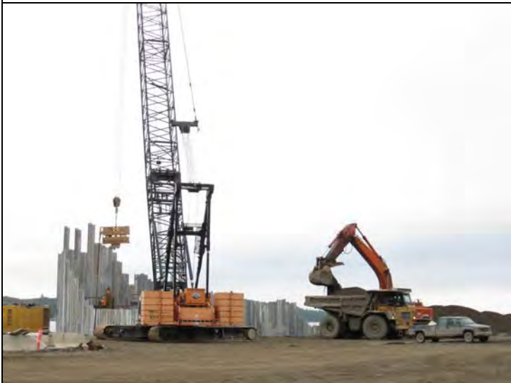
North pad, South End upon arrival – 2500 Orange finished driving sheets tail wall AA, Hitachi 700 trenches for extended tail wall
