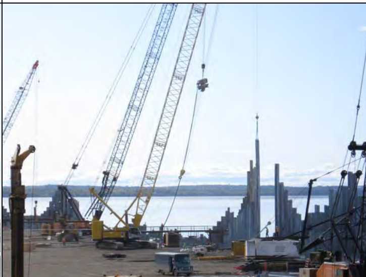
South pad, North end at departure – 2500 Orange returns Ape 200-6 towards cell 39 after setting down torn off sheet top
