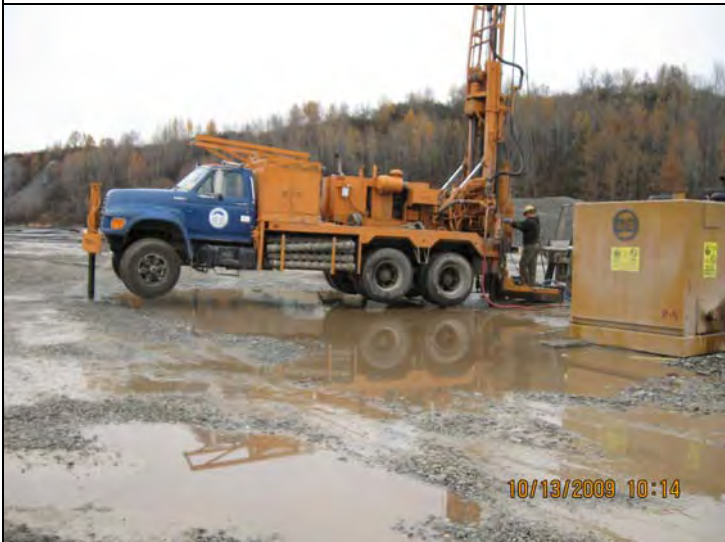
Denali drilling on site drilling SPT holes
