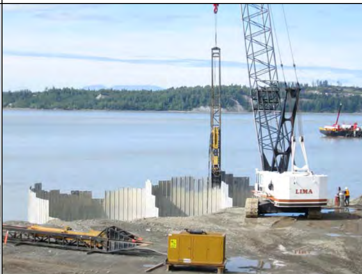
Wet Barge Berth at departure – White Sandstrom 'Lima' driving sheets w/ JM 115 impact hammer
