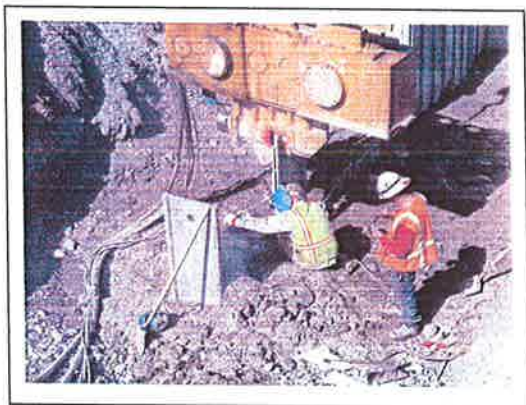
Figure 3 Welding sheets together so when a sheet is driven other sheets will not run
