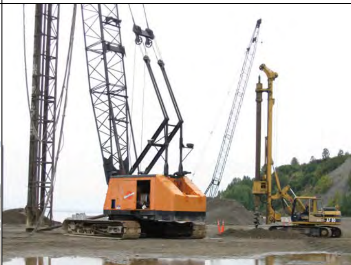
North pad, North End at departure – 4000w Vibe idle, Denali Drilling AF80 Auger boring holes in pad
