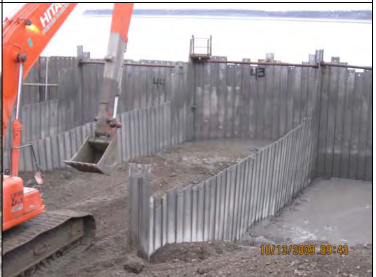
QAP excavator heading down cell 43 for silt removal,
