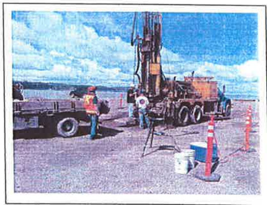
Figure 5 Predrilling for vibrocompaction
