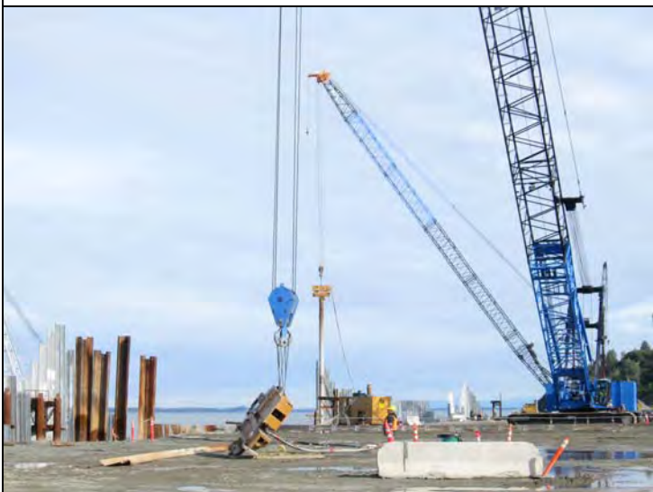
South pad, North end upon arrival – 2500 Blue picks Ape 200-6 in preparation for h-pile probing of problematic cells 38-39
