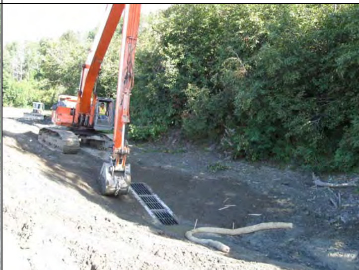
South Pad Drainage inlet – finished, covered up w/ cement cap and drainage grate, corps log installed, QAP Hitachi 450 finishing up grade – actively draining water in ditch
