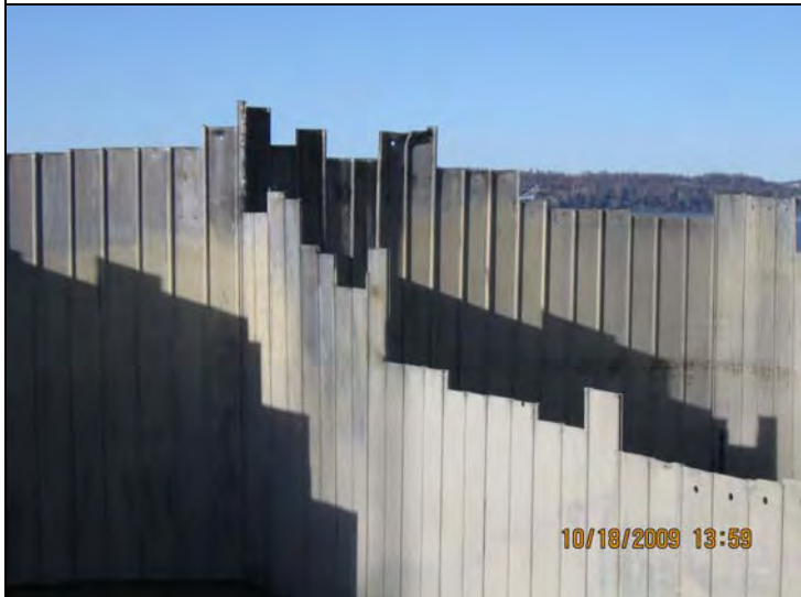
Wet Barge Berth cells 36&37 note recent fresh heading activities.
