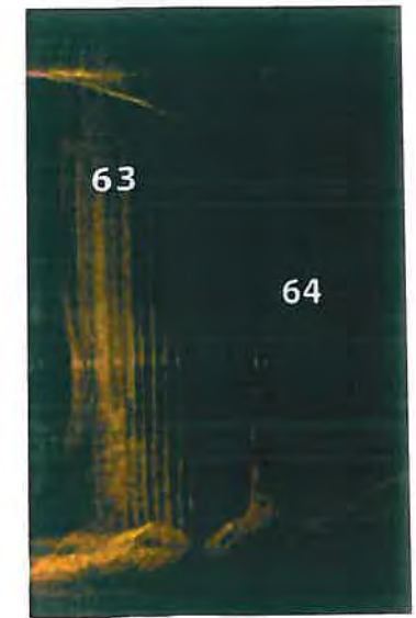
Interlocks on sheets appear to be straight and without gaps.
