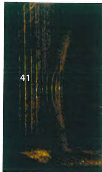
Interlocks on sheets appear to be straight and without gaps. The joints between 11 and 16 are visible on the sonar image.
