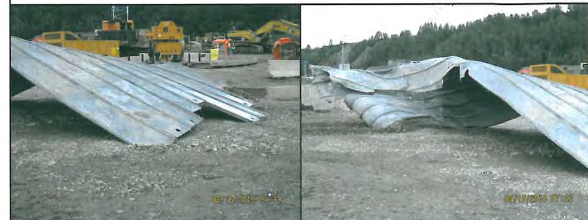
Cell 9 return cell sheets after pulling.
