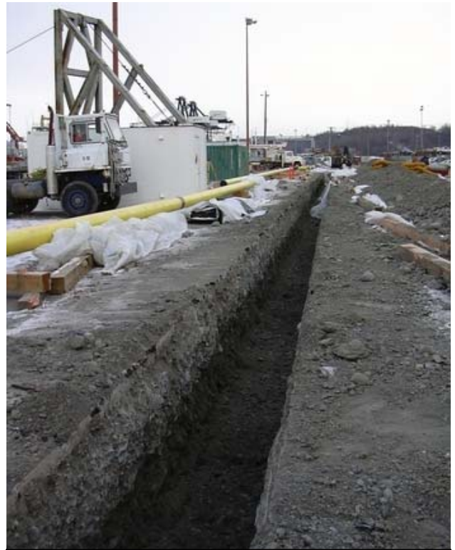
Fig 4: Dedicated low sulfur pipeline extension
