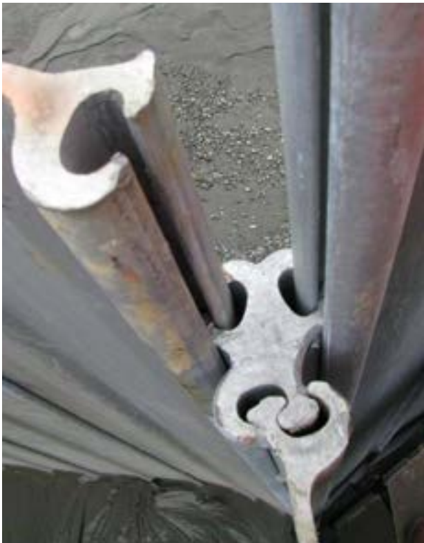
Fig. 2: Open Cell Sheetpile ® Foundation System
