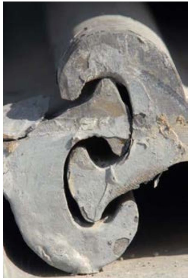
Fig 3: Sheetpile Interlock
