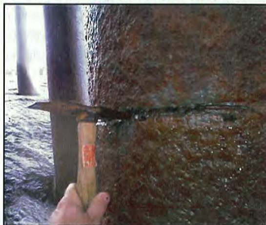
Figure 1-8 Pile Welds on a Corroding Pile
