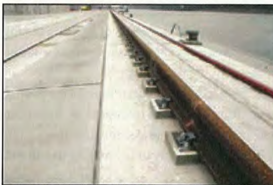
Figure 2-21 Waterside Crane Rail along Face of Dock
