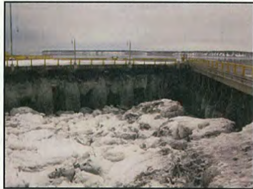
Figure 2-5 Ice around Pilings at the POA
